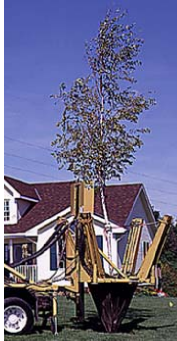
4--With the truck positioned near the hole, the tree is lowered into place, and the blades withdrawn.
